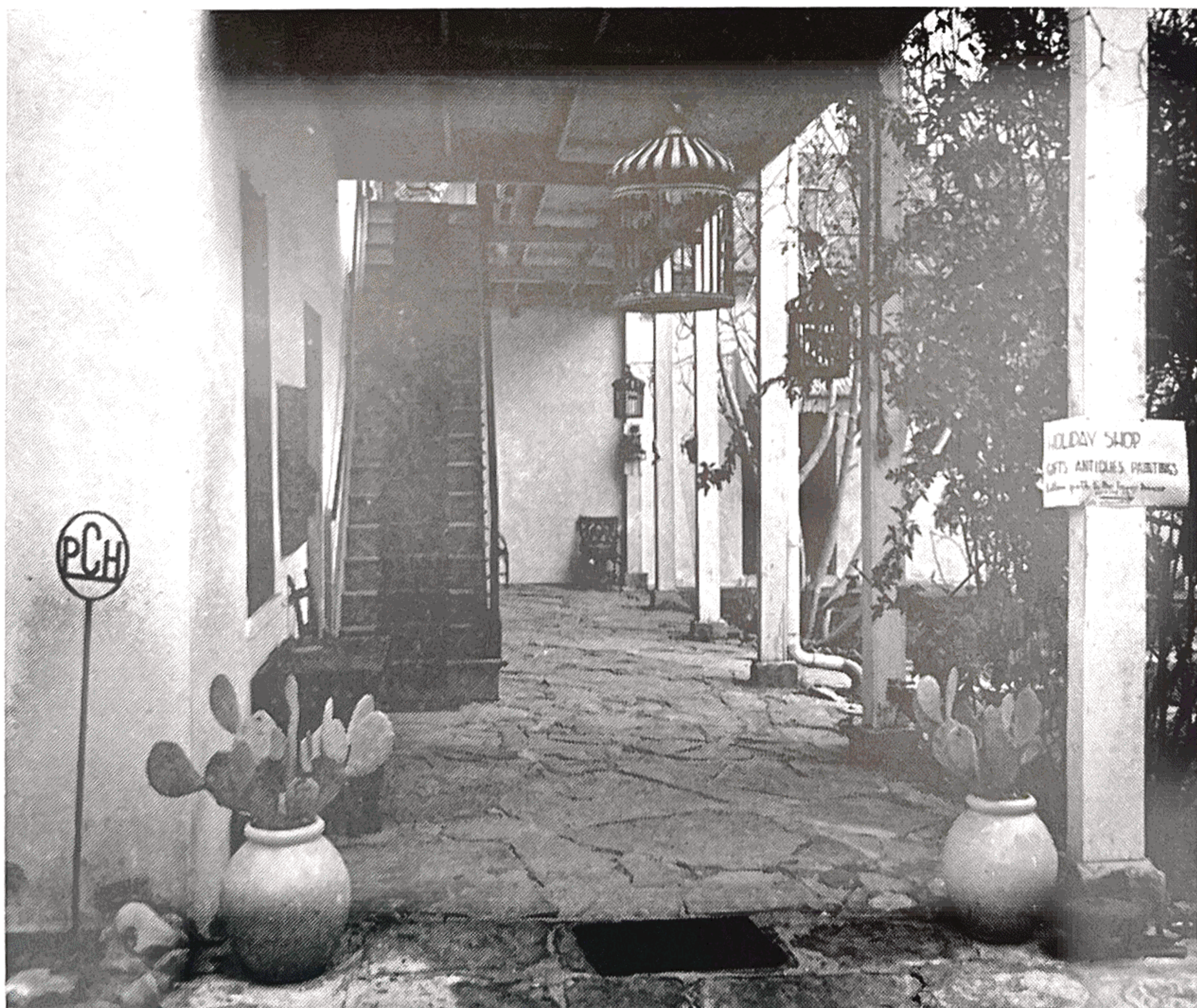
View of porch of Landmark Inn
